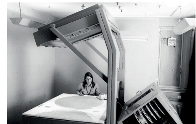
Figure 4: A “scanner” analyzes a bubble chamber photograph.
