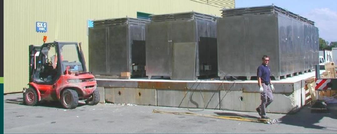
*Installation at Point 5 of the dump resistors for the CMS magnet surface tests.*
